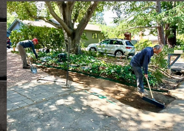
Driveway Driveway widened at street to facilitate full vehicle width. Dry well buried with valve.
