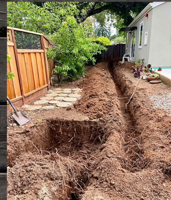
Move In! Comcast installed and a new punch list emerges.....electrical issues, vent issues, light issues, and trenches surround the house connecting all downspouts to a dry well below ground to hold rain water on site.
