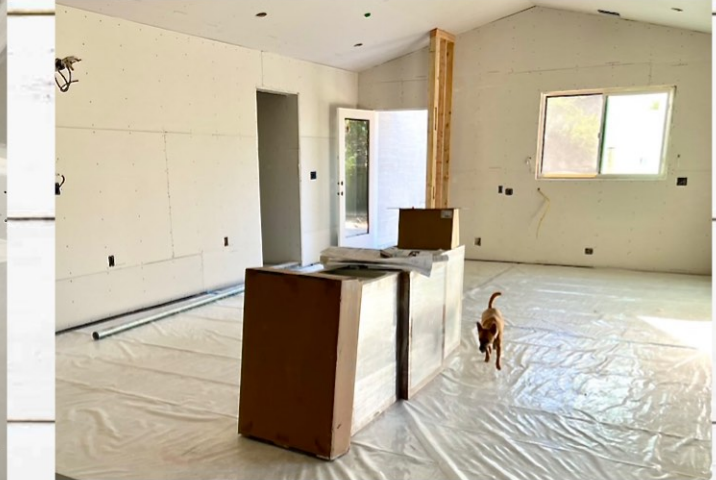
Wall Prep Mud inside. Second coat of stucco outside. RedGuard in bathrooms for waterproofing. Orange under heated flooring.
