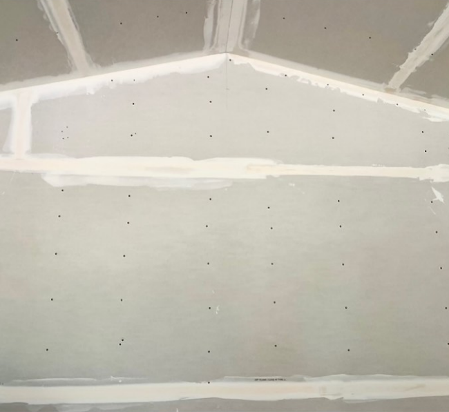
Wall Prep Mud inside. Second coat of stucco outside. RedGuard in bathrooms for waterproofing. Orange under heated flooring.
