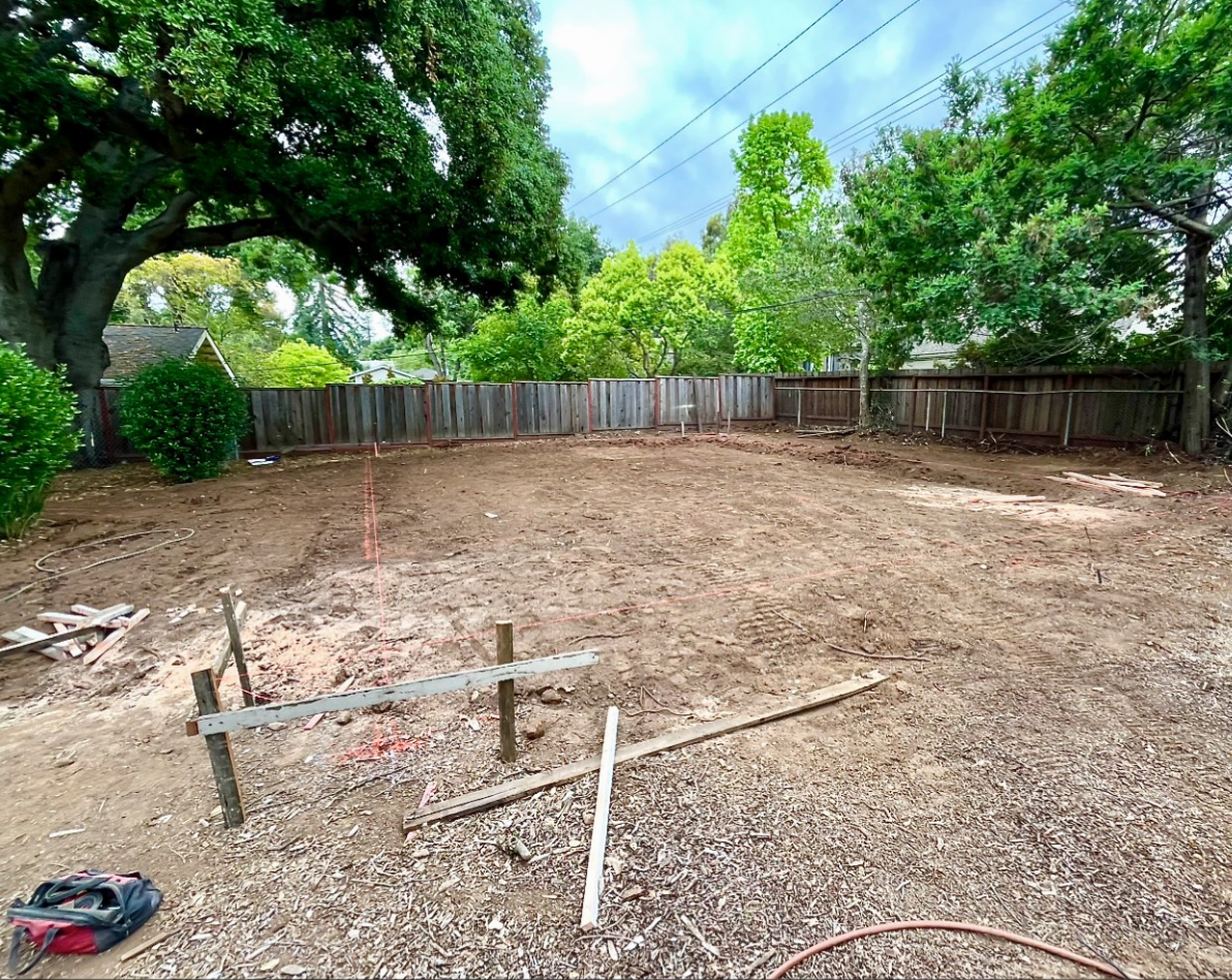
Prep A clean slate emerged. The ground was leveled, forms made, plumbing installed, gravel and rebar applied for strength and the foundation was ready to be poured.
