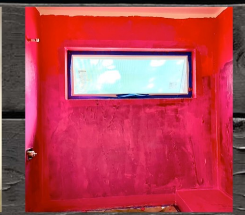
Wall Prep Mud inside. Second coat of stucco outside. RedGuard in bathrooms for waterproofing. Orange under heated flooring.
