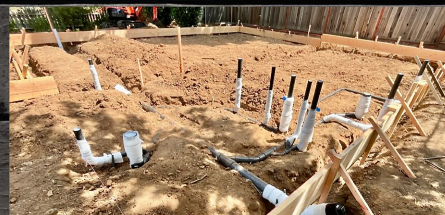
Prep A clean slate emerged. The ground was leveled, forms made, plumbing installed, gravel and rebar applied for strength and the foundation was ready to be poured.
