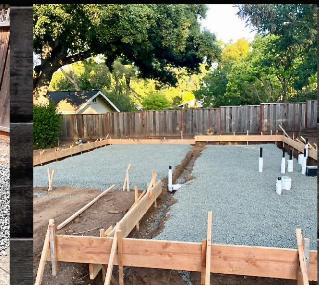
Prep A clean slate emerged. The ground was leveled, forms made, plumbing installed, gravel and rebar applied for strength and the foundation was ready to be poured.
