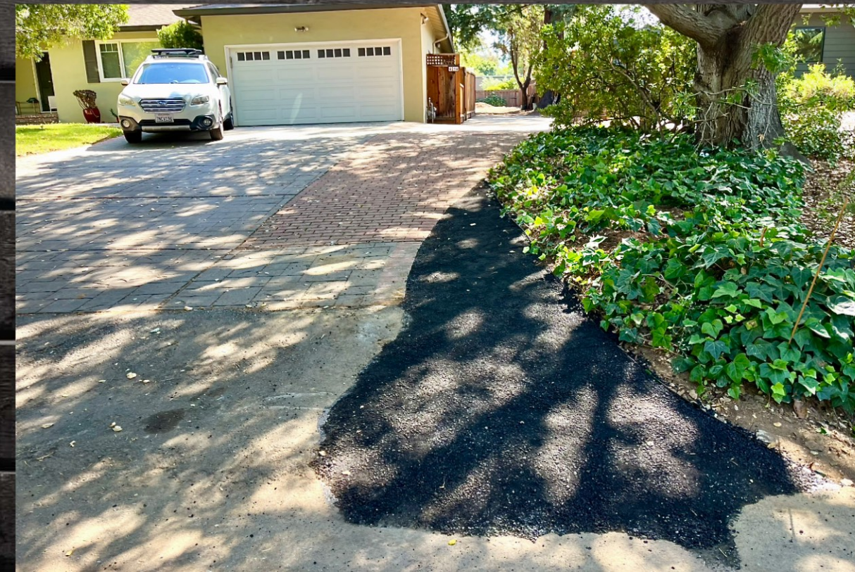
Driveway Driveway widened at street to facilitate full vehicle width. Dry well buried with valve.
