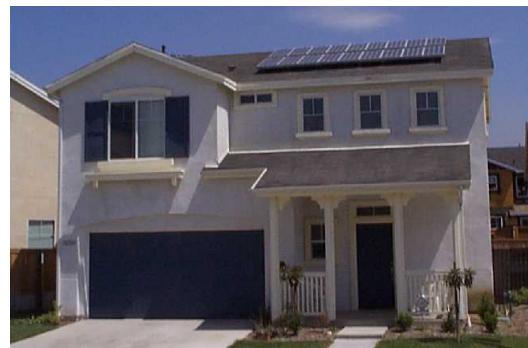
Figure 1 Roof Mounted PV System
