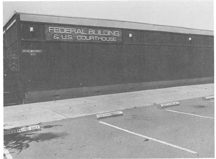
The temporary Federal Building and United States Courthouse on West Taylor Street in San Jose. This view shows the judges’ parking area on the northeast side of the courthouse building. (Photograph by Ira Nowinski.)
